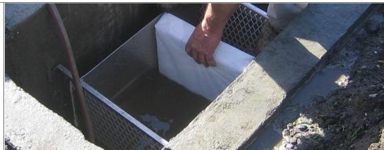
The Smart Pak is designed for use in new or existing stormwater vaults that experience hydrocarbon, heavy metal pollution accompanied by sediment, debris, or bacteria. Smart Paks help meet or exceed stormwater National Pollutant Discharge Elimination System (NPDES) permit requirements with effective filtration, absorption, life expectancy, and maintenance costs.
